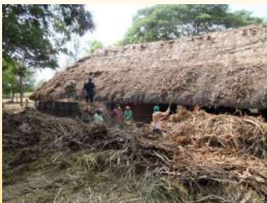
Taking down the thatch roof
