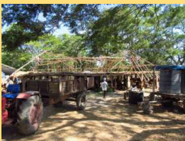
Taking down the wood structure
