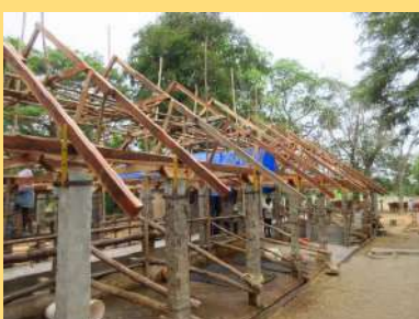
carpentry work for the new structure
