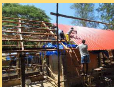
Adding the roof sheets
