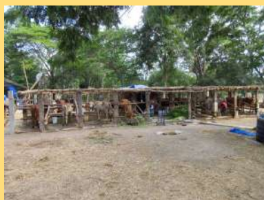
without roof structure
